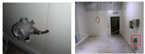
Figure 4. Leak detection sensor and location inside Climatic chamber.
