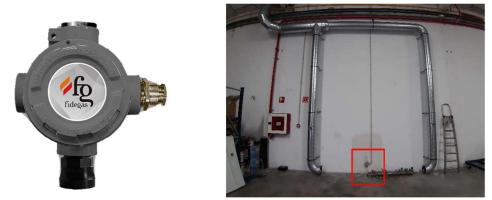
Figure 3. Leak detection sensor and location in Charging zone prepared with the air extraction system.
